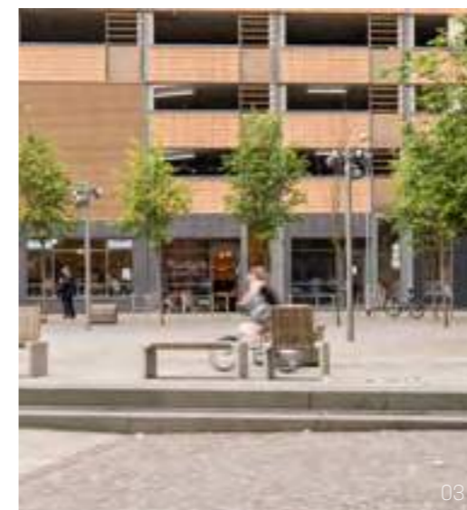
03 | Multi-storey car parks on the periphery of the city
