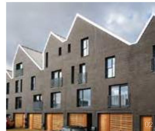
02 | Sustainable design that is solar efficient
