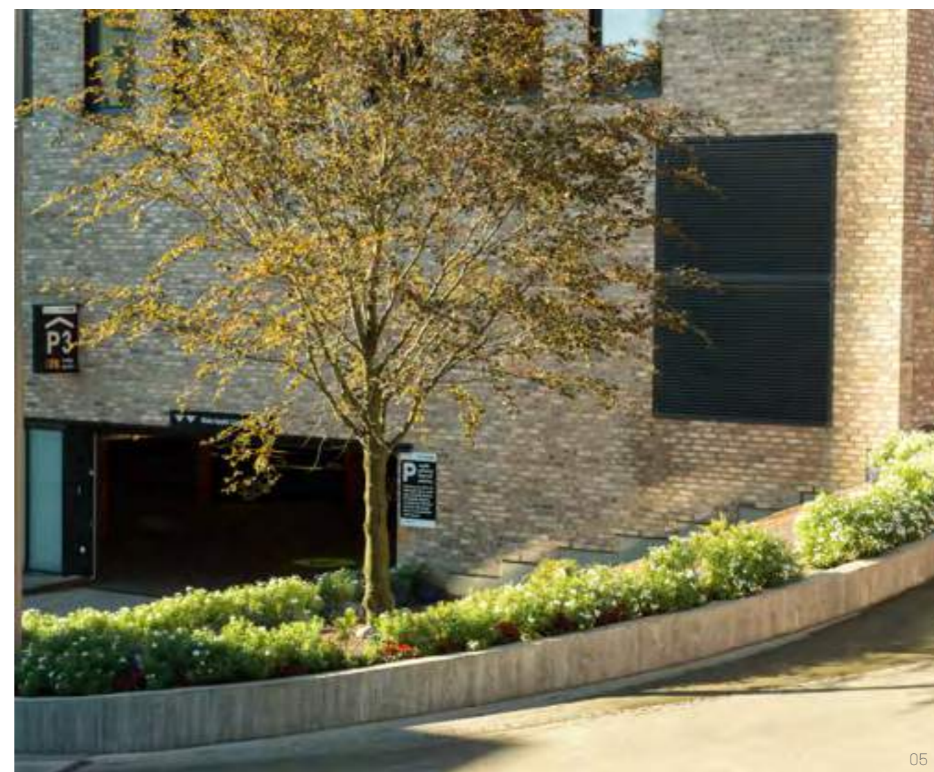
05 | Underground car parking
