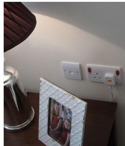
The specification of internal fittings and fixtures is important in making extra-care dwellings accessible but not institutional (image: Swallowdale Extra-care, Edlington).
