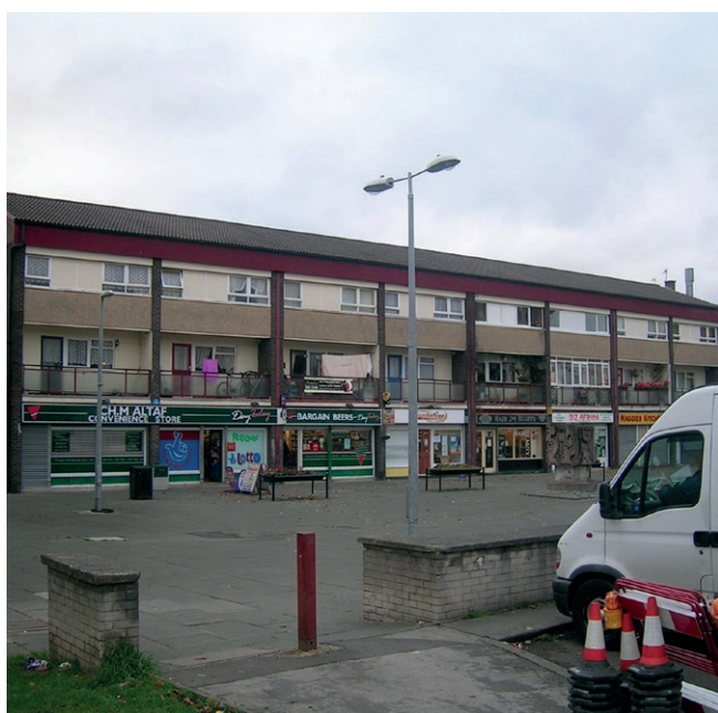
Eastford Square in Collyhurst, which is now derelict and awaiting demolition Source: Flickr / Raver_Mikey
