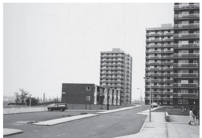
1960's Radburn housing and tower blocks Source: Manchester Libraries, Information and Archives
