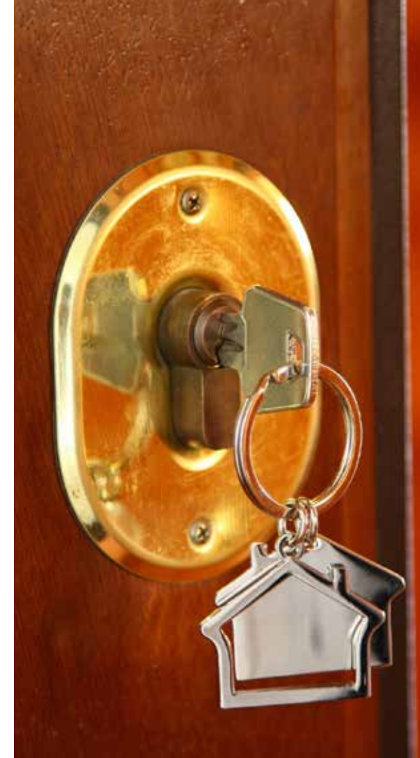
Raised keyhole in colour which contrasts with door
